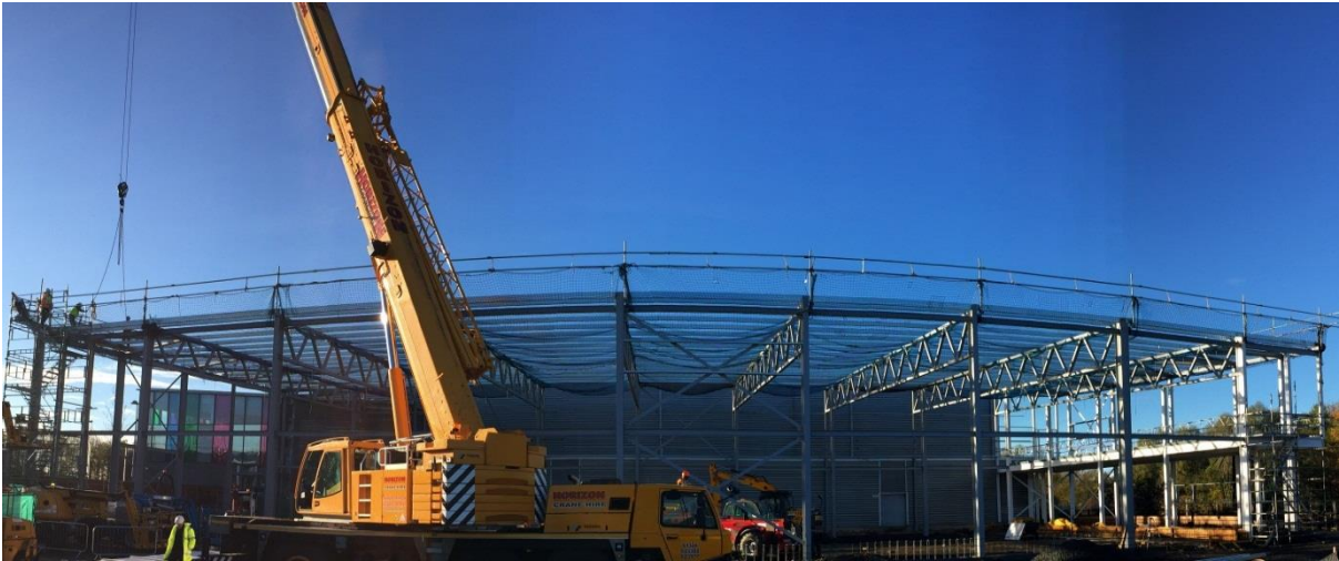
[National Curling Academy construction site Nov 2016]
